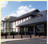
West Cornwall Hospital, Penzance
